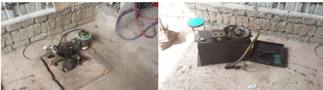
Fig No.3 .Disassembled Hydraulic Power Pack.
